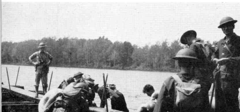
Foot bridge at Macomb Reservation.
