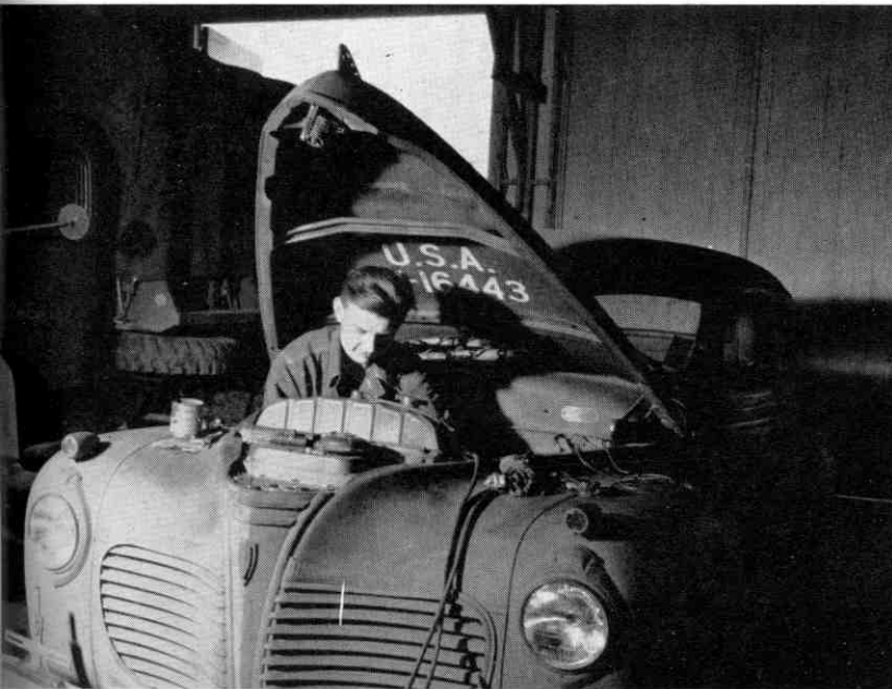
Repairing power unit.
