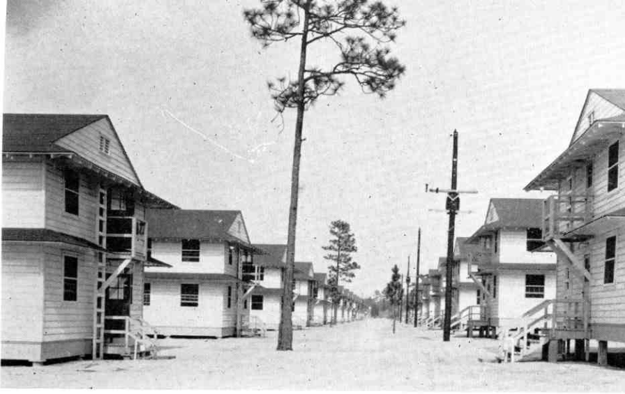
ENLISTED MEN'S BARRACKS
