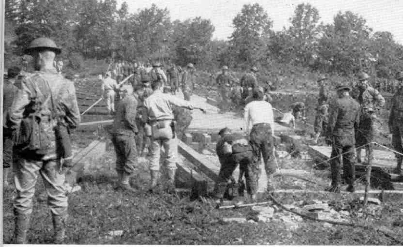
Constructing Ponton Bridge on Saranac River.
