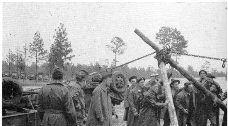
Adjusting and tightening a prone for righting overturned truck.
