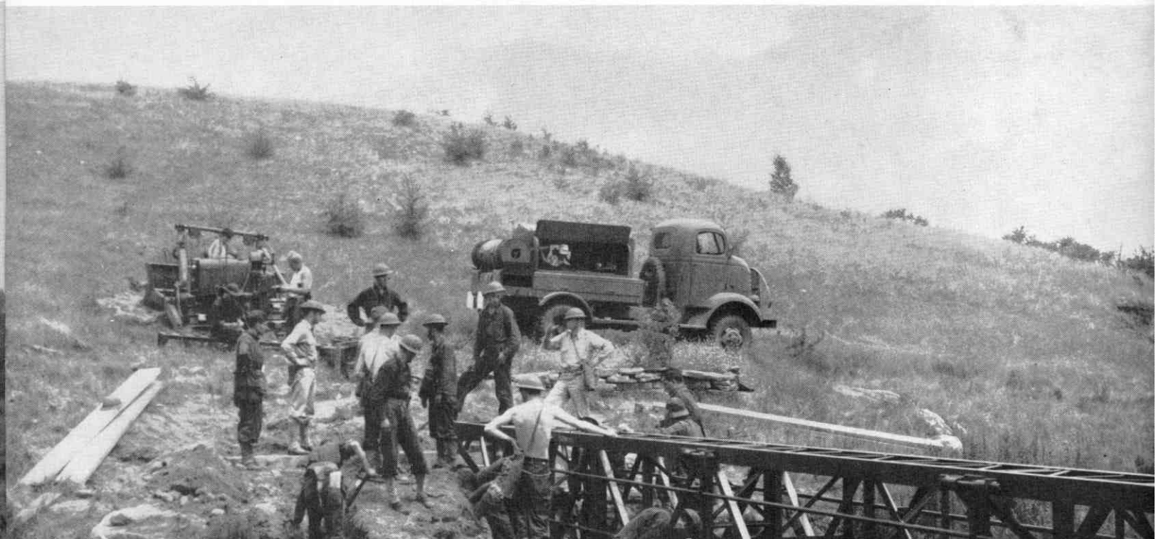
H-10 bridge being assembled over ravine.
