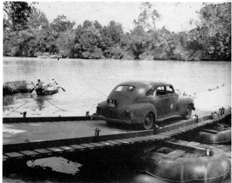
Official car crossing rubber ponton bridge at Leahs Ferry.
