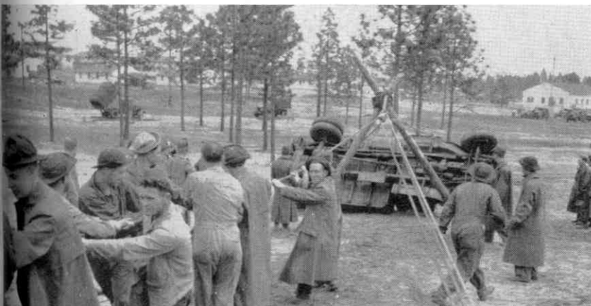
Heaving on block and tackle to right overturned vehicle.
