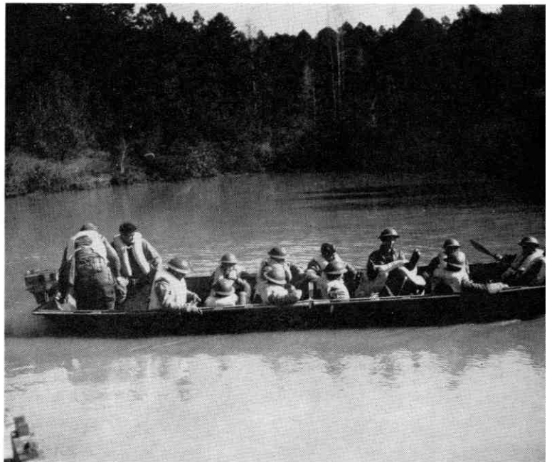
Powered storm boats take the Engineers across to destroy the enemy.
