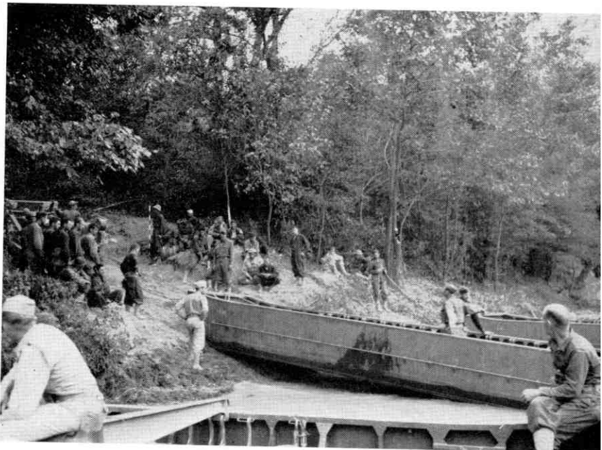
Removing ponton from river by use of Angle Duzer.
