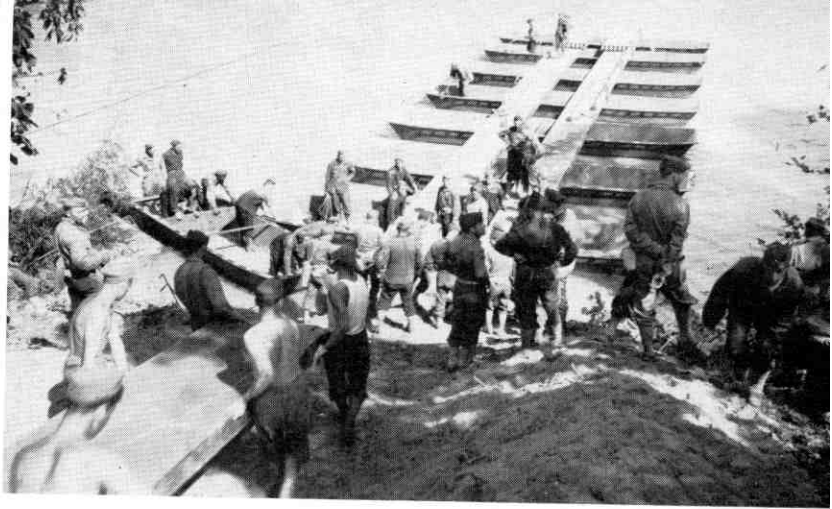
Constructing half boat bridge over Pee Dee River.
