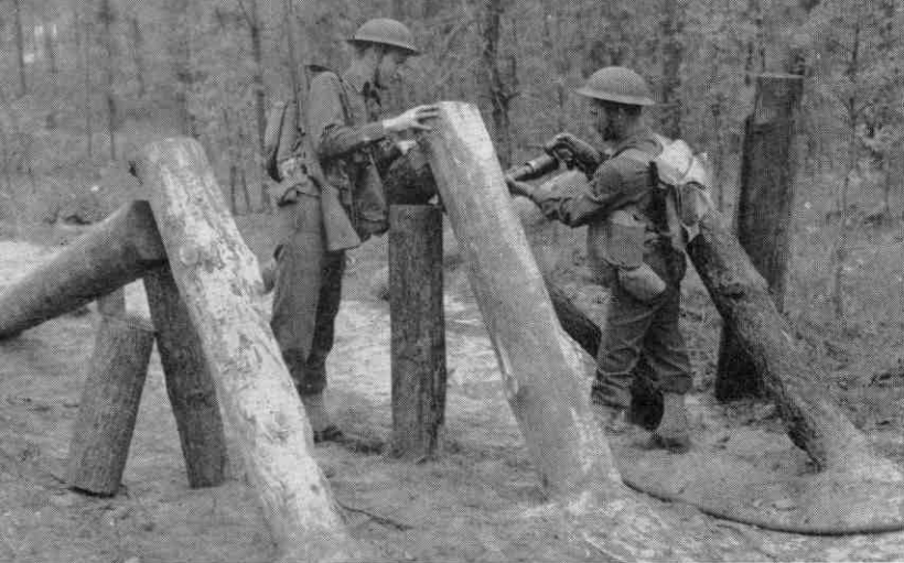
The 36th Engineers constructing road block using pneumatic hammer.
