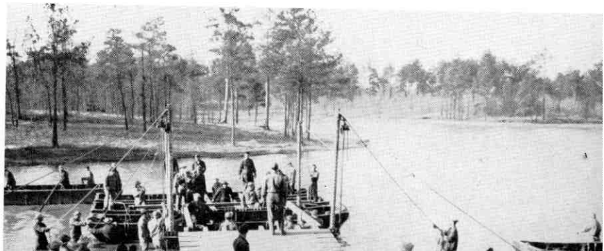
General view of bridge over Mac Faydens Pond.
