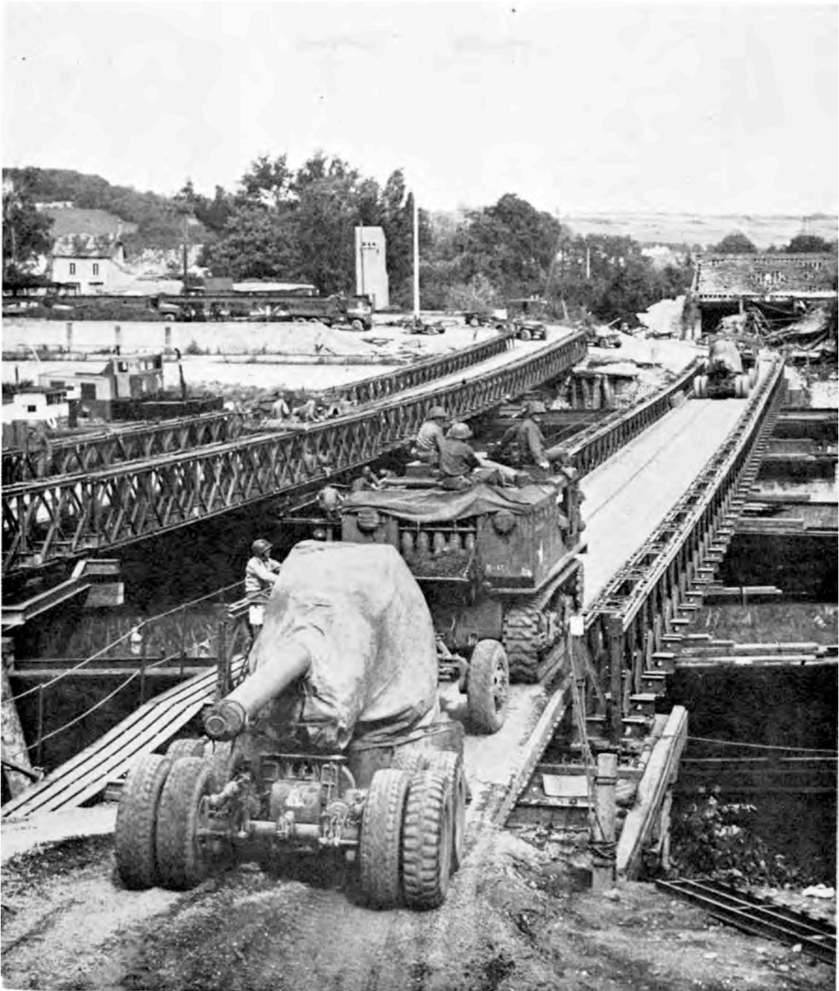
During the Battle of the Bulge, the 631st helped build floating Bailey bridges over the Meuse River in Belgium, similar to this one over the Seine in France. ( Corps of Engineers: War against Germany , 193.)
