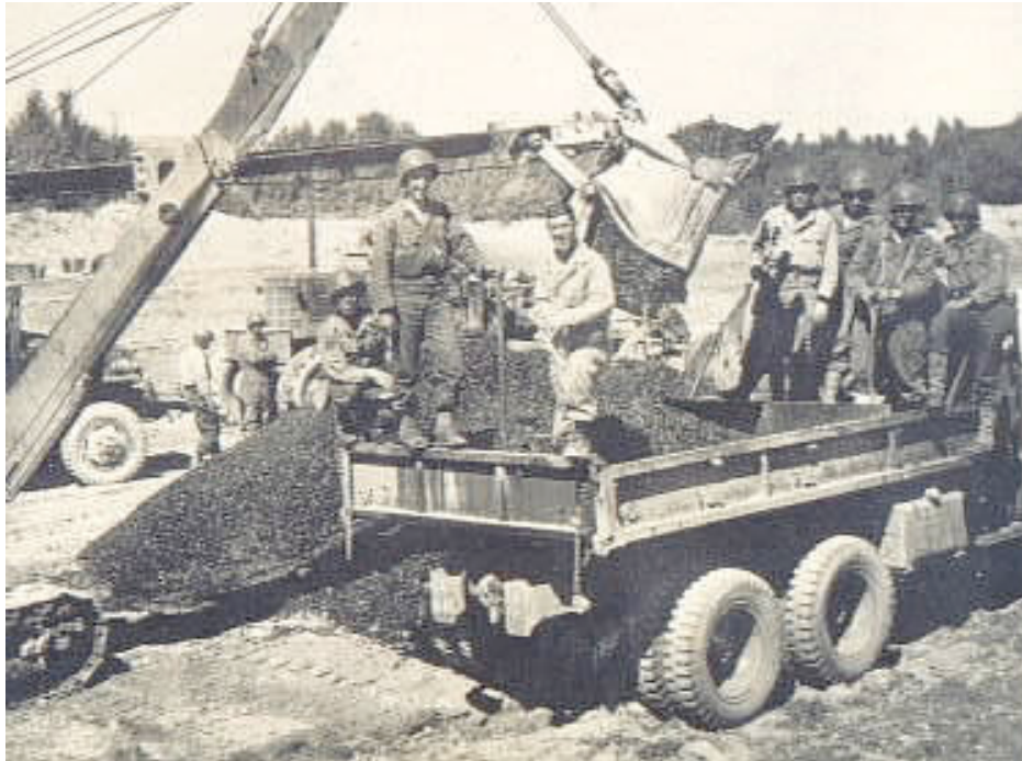
At a 631st rock quarry, a crane operator drops gravel into the bed of a dump truck. Bill Kepp stands in the truck bed at center foreground. (Courtesy Deborah Fiducia.)
