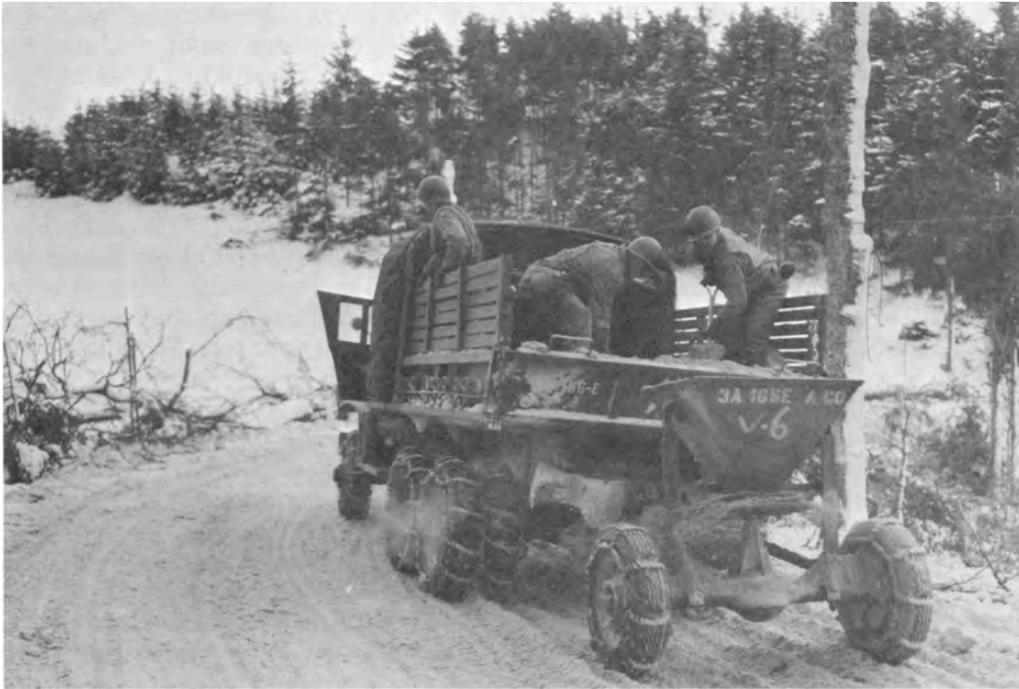
Engineers shoveling abrasive materials onto a road outside Wiltz, Belgium, during the winter of 1944–45. ( Corps of Engineers: War on Germany , 477.)
