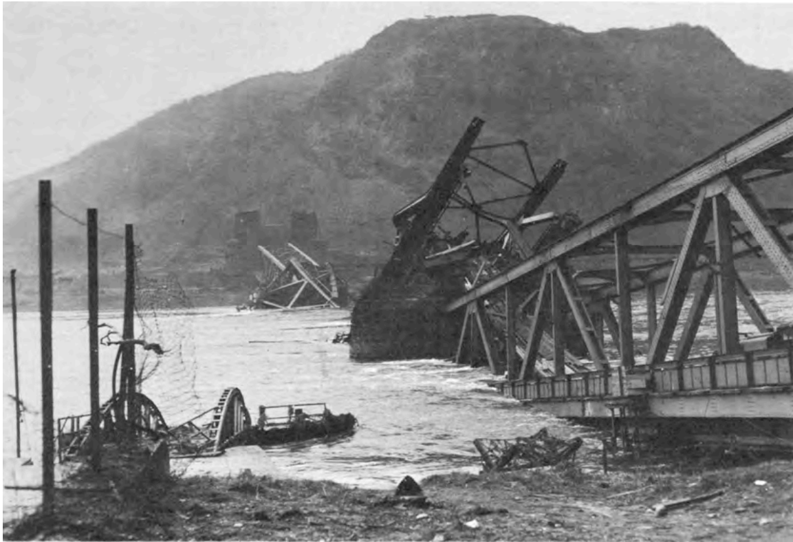
Wreckage of the Ludendorff railroad bridge after its collapse on March 17, 1945. ( Corps of Engineers: War on Germany , 512.)
