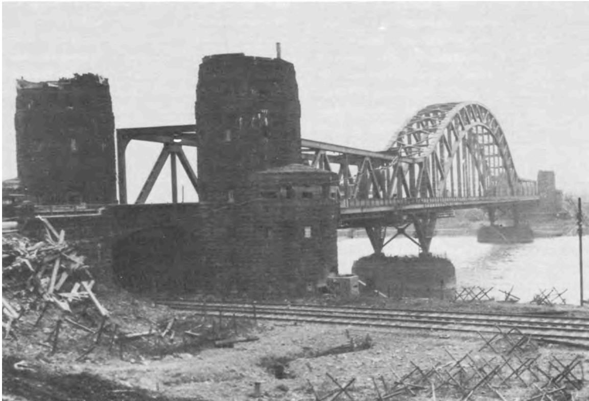
The Ludendorff railroad bridge across the Rhine at Remagen. By the time this photo was taken, traffic across the bridge had been halted while engineers worked on repairs. ( Corps of Engineers: War on Germany , 501.)
