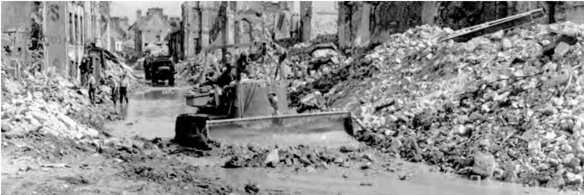
An important job for engineers throughout the war in Europe was clearing streets in bombed cities, to keep Allied forces moving through them. Here, a driver bulldozes rubble in Cherbourg, France, 1944. ( War against Germany , 129.)
