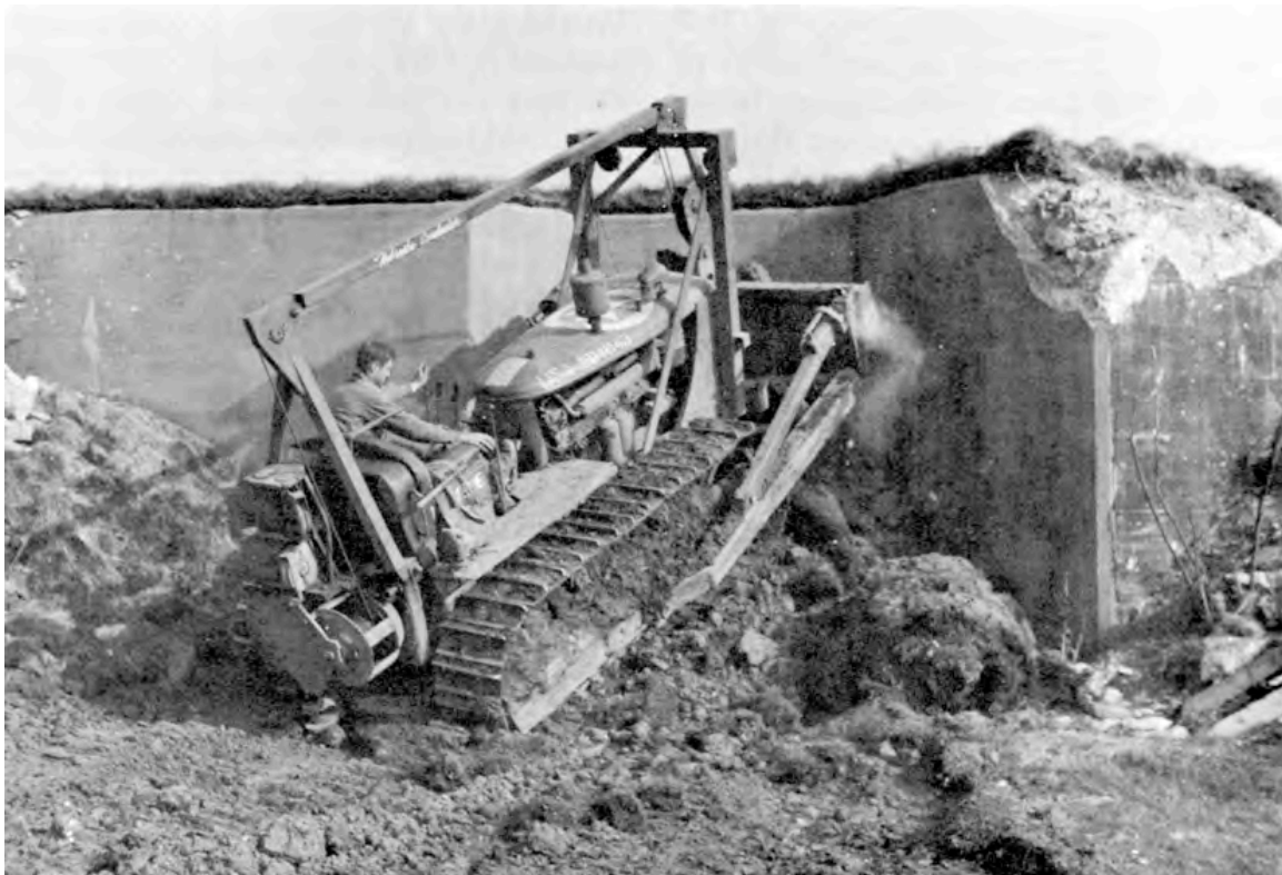
A bulldozer operator seals German bunkers in the West Wall outside Aachen, Germany, 1944. ( Corps of Engineers: War on Germany , 419.)
