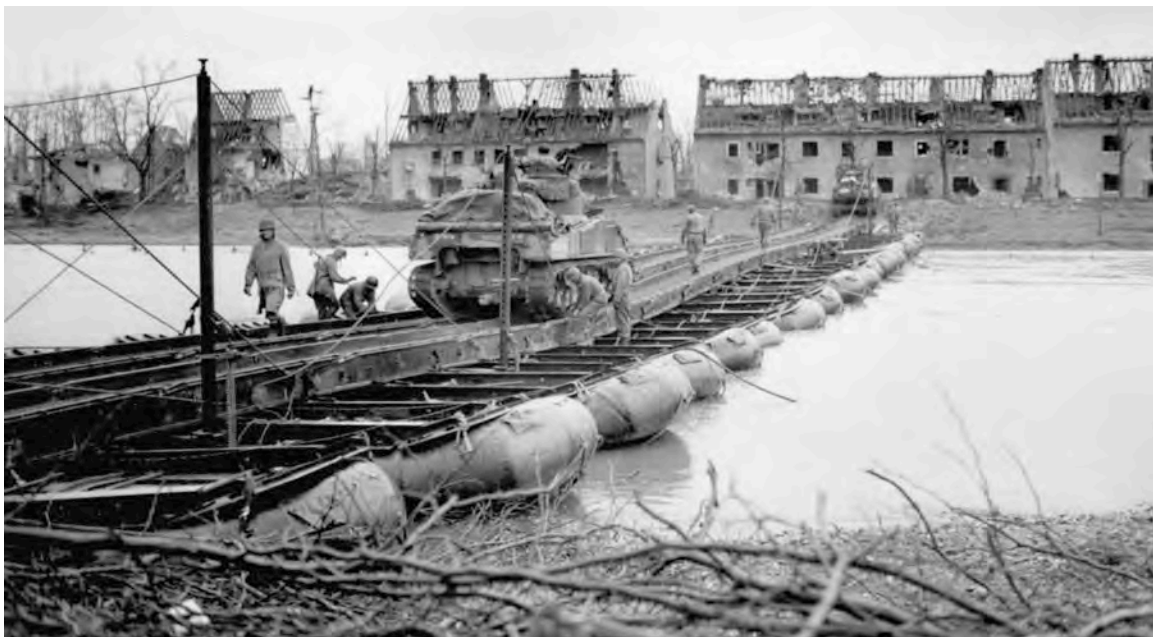
Tank crossing the Roer on a pontoon treadway bridge, February 1945. Shelled buildings stand on the far shore. ( Core of Engineers: War against Germany , 340).
