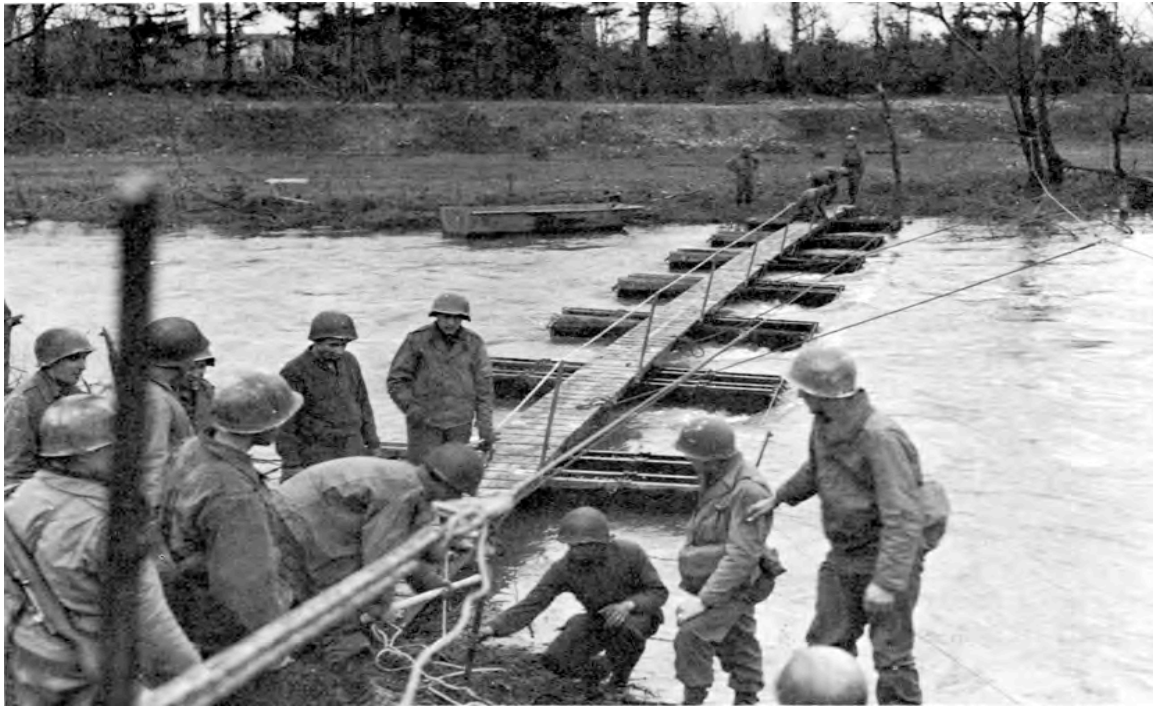
Engineers attaching the cables of a pontoon-supported foot bridge across the Roer River, February 1945. ( Corps of Engineers: War against Germany , 498.)
