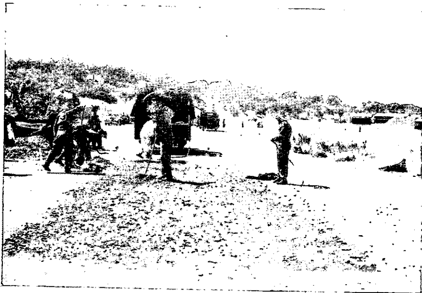
FIGURE 73.—Texturing runway with wood chips to produce darker tone from the air and reduce contrast with surrounding area.
