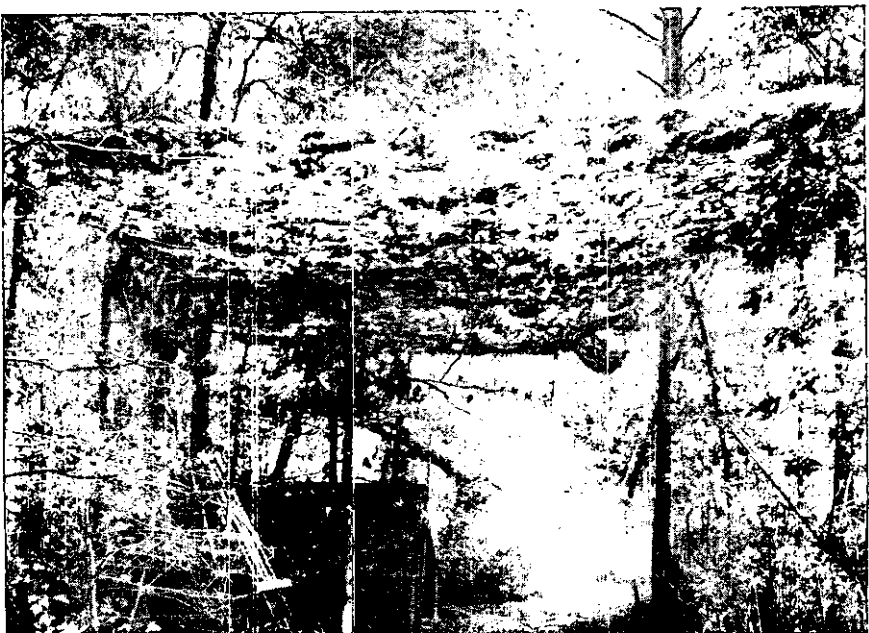
FIGURE 70.—Overhead screen conceals short stretch of access route.
