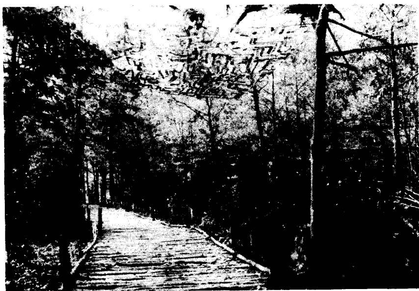
FIGURE 30.—In a more permanent location, short stretches of a newly made, much-used road may be covered by an overhead screen made of wire and cloth garnishing material. Notice tops of trees tied together in background.
