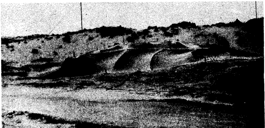
FIGURE 52 ① and ②.—Drapes, placed to resemble surrounding terrain, cover headquarters in desert. Note compact assembly of vehicles under framework being erected to simulate mound shown below. Installation is effective against both direct and photographic observation. This is a necessary exception to dispersion; vehicles are dispersed by groups rather than by individual vehicles.
