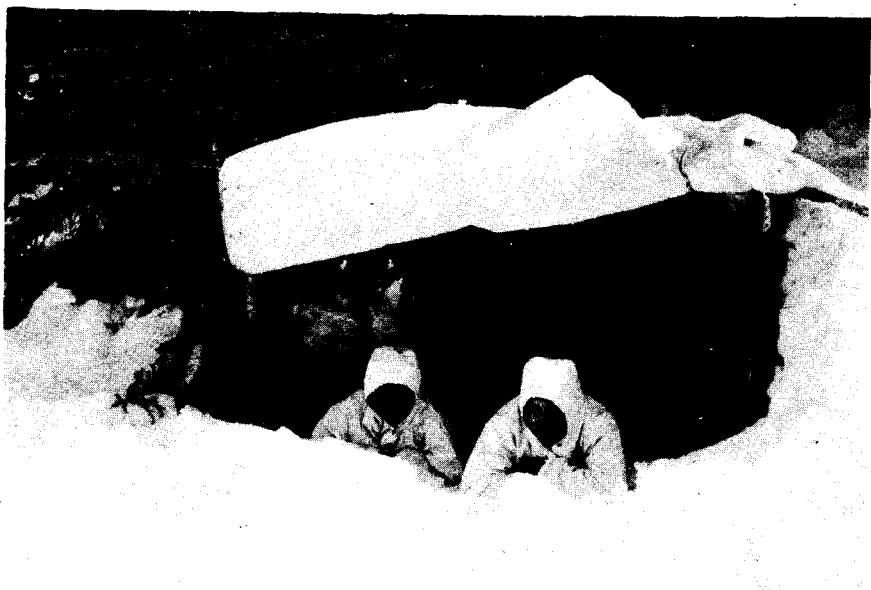
FIGURE 24.—Shelter halves painted white and used in conjunction with post supports and natural materials to provide shelter and concealment. Trees and branches placed around the outside of the structure aid in camouflage. Whenever possible pile snow irregularly around tents and other objects to aid in blending.
