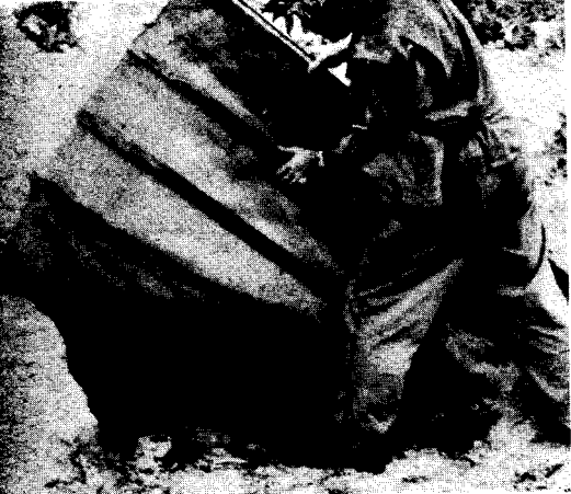
FIGURE 69 ① and ②.—An embankment is a convenient place in which to dig in supplies. Here an excavation has been made, supplies laid in, and the opening covered with cloth reinforced with slats. Pit with cover on is almost invisible, even to the ground observer.
