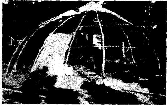
FIGURE 71 (b).—Thatching is laid on in sections. Attach hay to cloth base by means of an adhesive. Sections are wired to frame.
