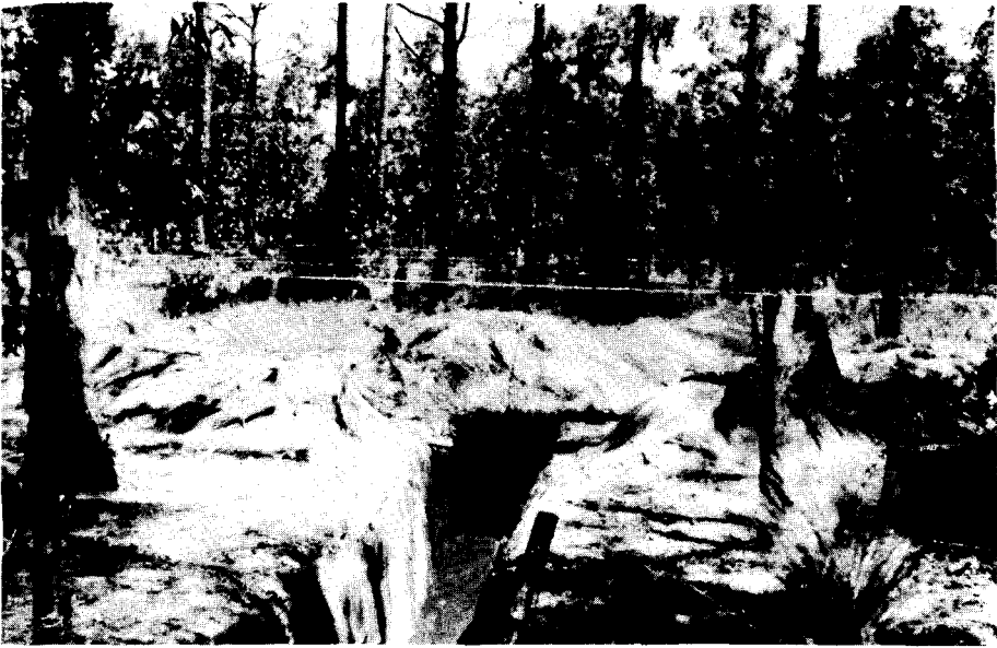
FIGURE 74 (a) and (b).—Supply trenches, sited in woods with insufficient overhead cover, being concealed with flat-top. Net is erected before digging is begun. In above photo, net has been removed to show details. Below, with garnished twine net in place, shadows of trenches are broken up.
