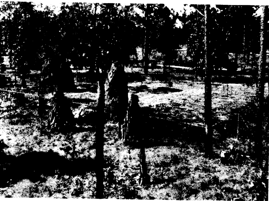
FIGURE 74 (c) and (d).—Above, view showing excellent matching texture achieved by well-garnished flat-top over supply trenches in (a) and (b). Below, completed job, with imitation trees made of chicken-wire cones garnished with artificial materials and sited to break up what shadows remain at edge of net.
