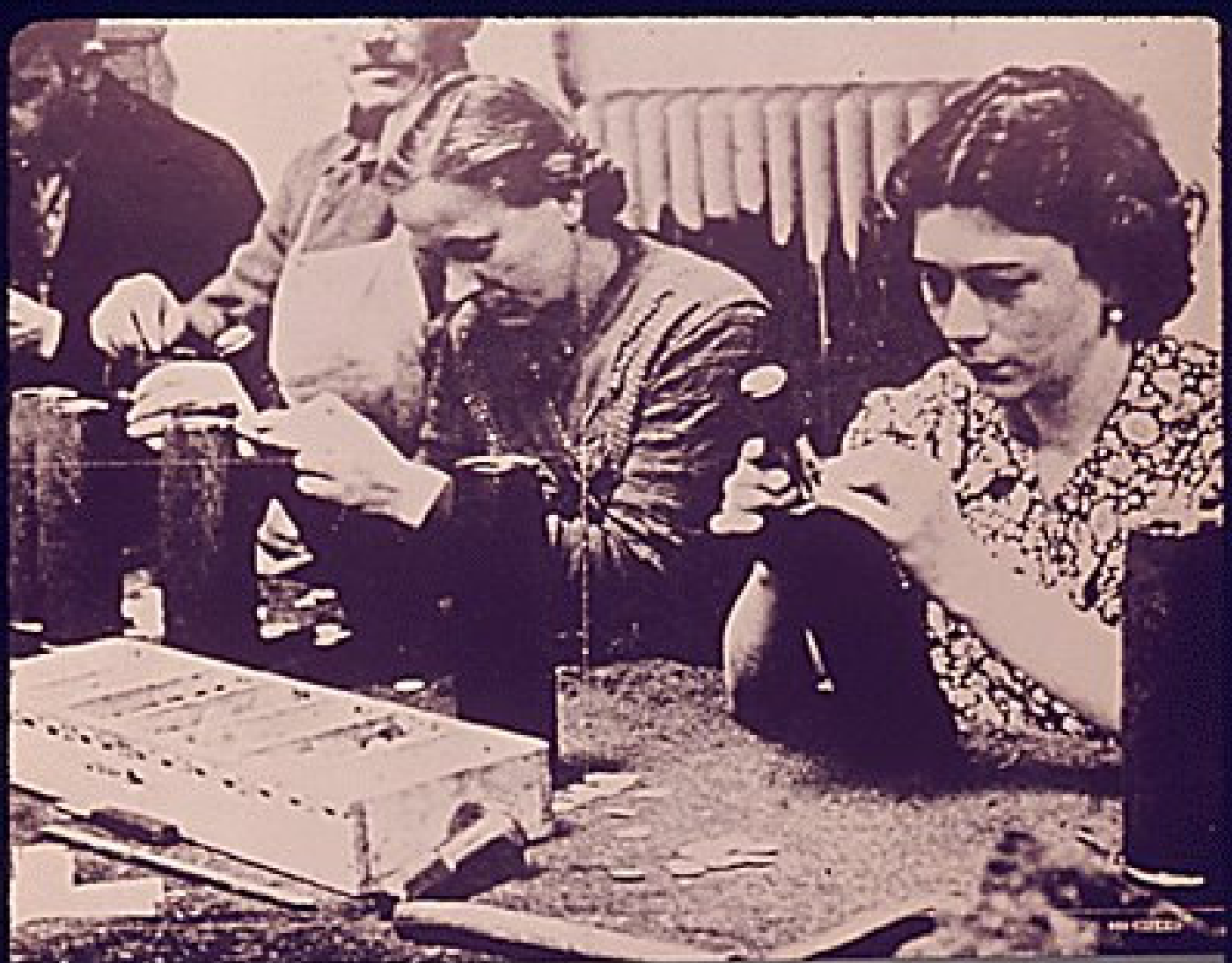
THIS PHOTO, TAKEN SECRETLY, SHOWS WORKERS IN A NAZI WAR PLANT
