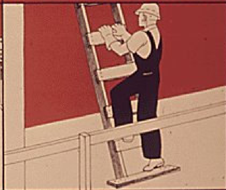
NAIL IN PLACE ON CONSTRUCTION JOBS
