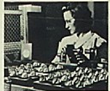
ALIGNING PRISMS FOR BINOCULARS
