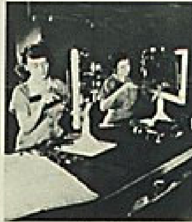
INSTALLING INSTRUMENTS ON BOMBER INSTRUMENT PANELS
