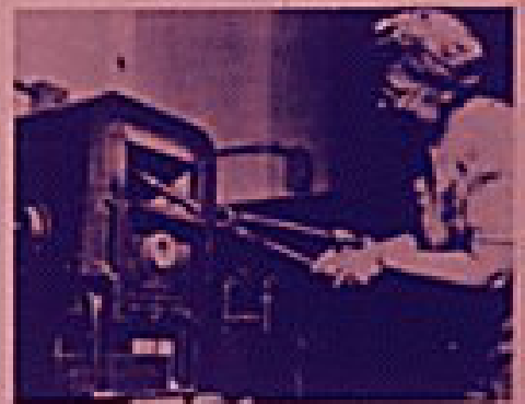
LABORATORY ASSISTANT TEMPERING METAL IN GAS FURNACE
