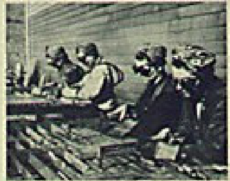
SHIPYARD BURNERS CUTTING METAL PLATE WITH ACETYLENE FLAME
